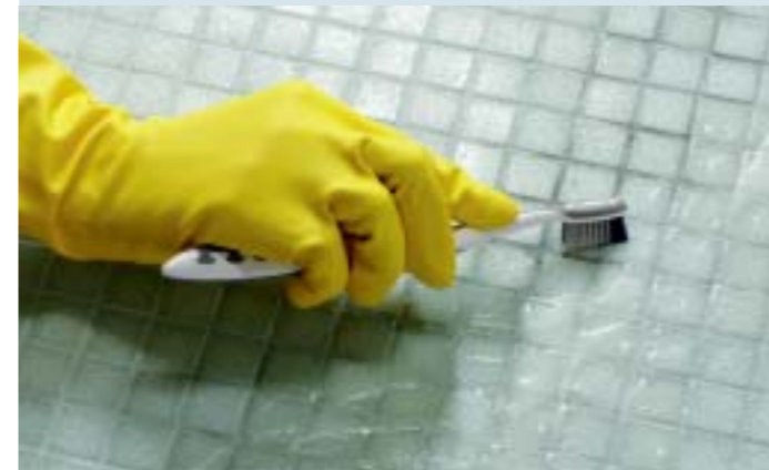
Tiled shower areas need work-intensive cleaning.
